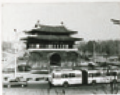
THE TOWER OF THE GREAT WALL
