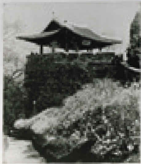
THE TOWER OF THE GREAT WALL
