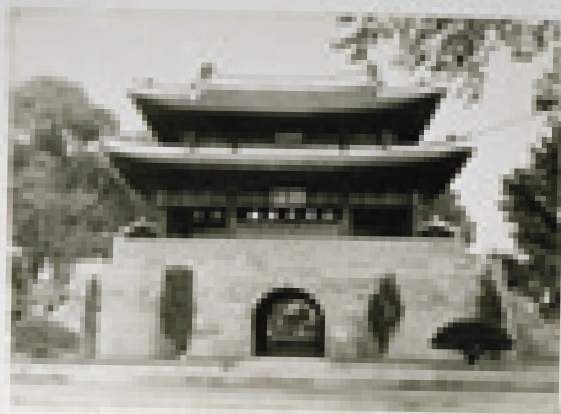
THE TOWER OF THE GREAT WALL
